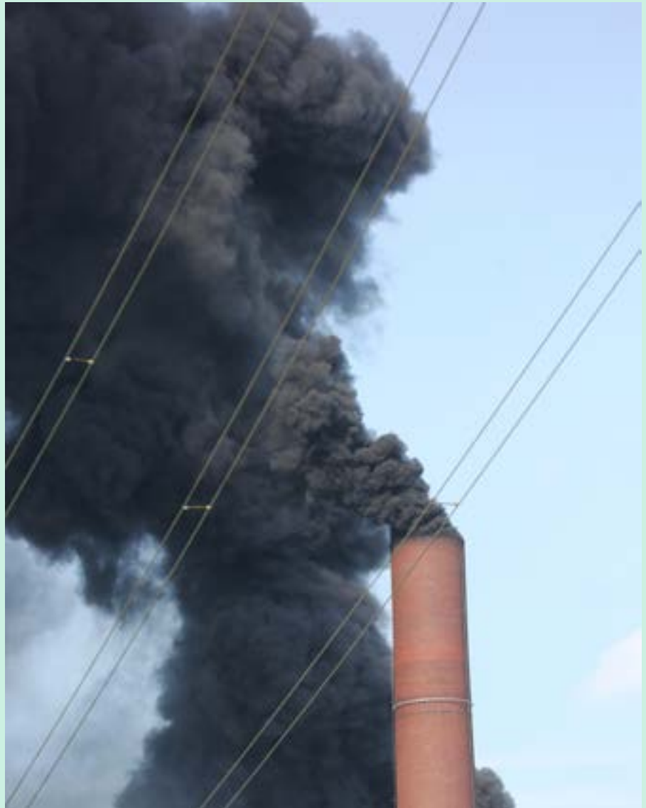
Shell Refinery Wesseling
