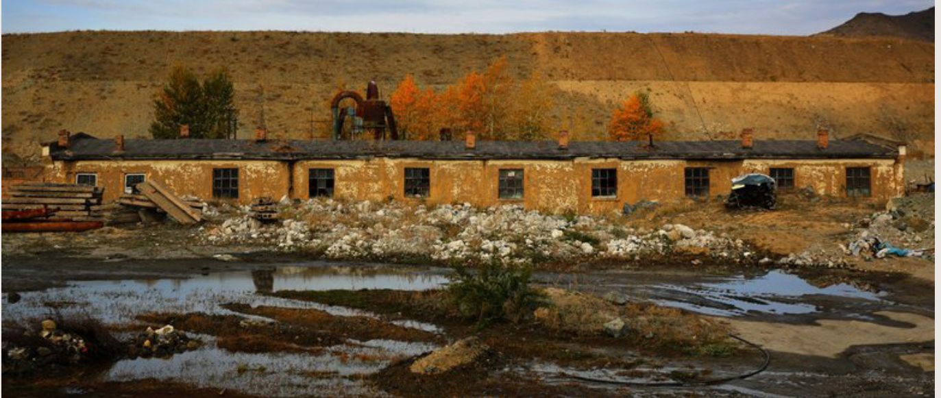
A view of the No.3 Pit mine in Fuyun or Koktokay county, Altay Prefecture, northwest China's Xinjiang Uyghur Autonomous Region,
